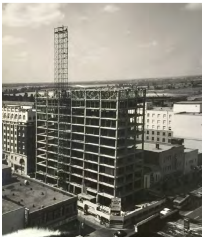
Above: Petroleum Tower under Construction, 1957. Right: Postcard of the Henry C. Beck Building, ca. 1950s. Sources: Downtown Development Authority, eBay.
